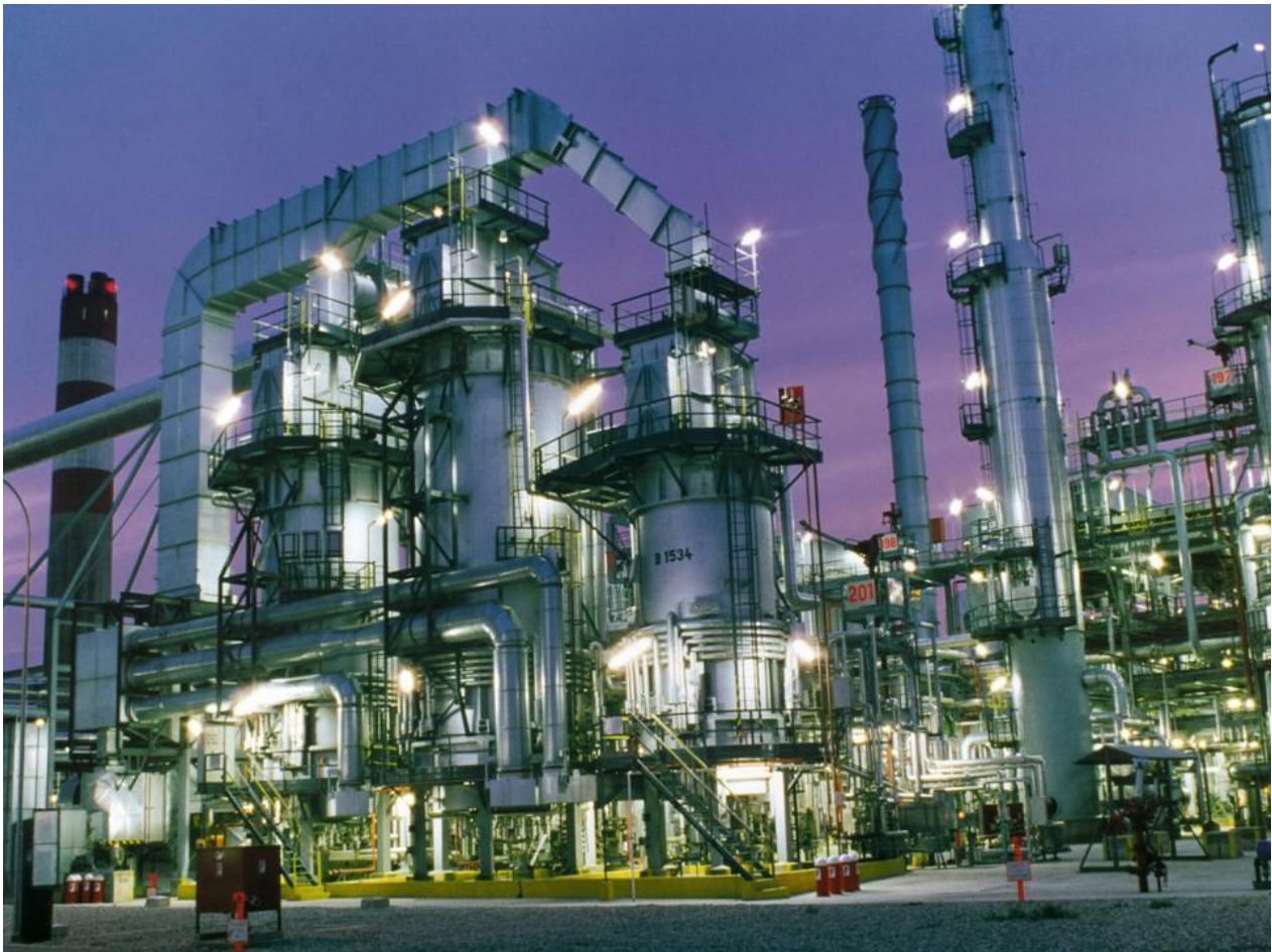
Oil Refinery Plant
