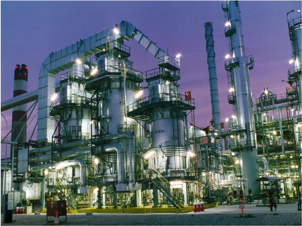
Oil Refinery Plant
