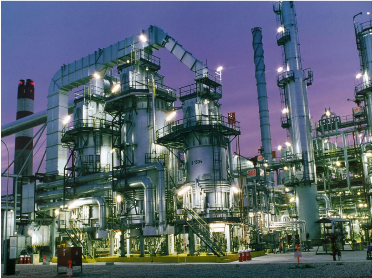
Oil Refinery Plant
